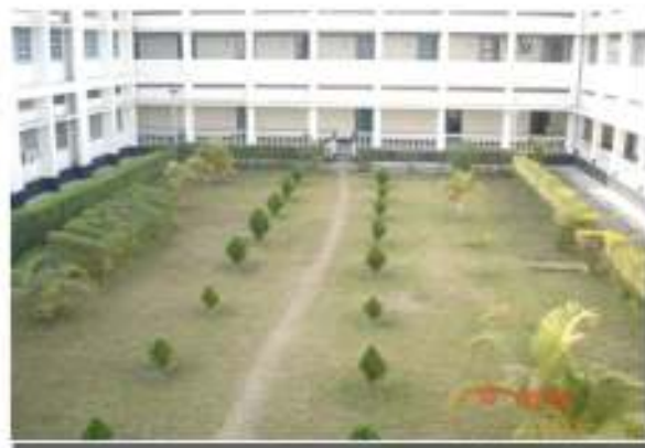
A view of the administrative block
